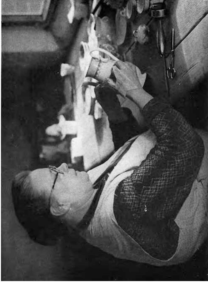
The Transferrer cuts up the tissue transfer and applies it face downwards to the portion of the article to be decorated, rubbing it down into optical contact with a stiff brush. The paper is afterwards washed off, leaving the design on the ware. Great accuracy is needed in the application of the transfer.
